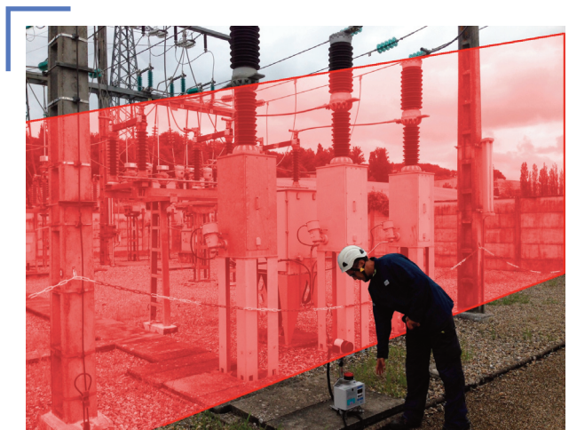
Work in a substation
