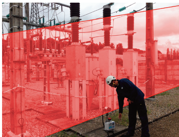
Work in a substation
